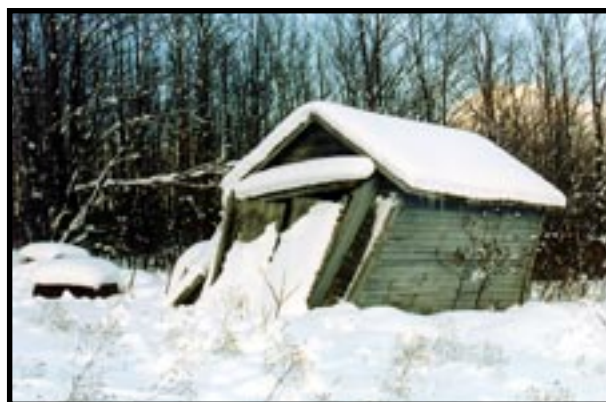
The old garage is strained by the weight of too much snow.
